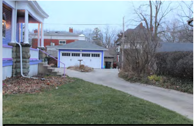
PARTIAL NORTH SIDE & GARAGE EAST SIDE
