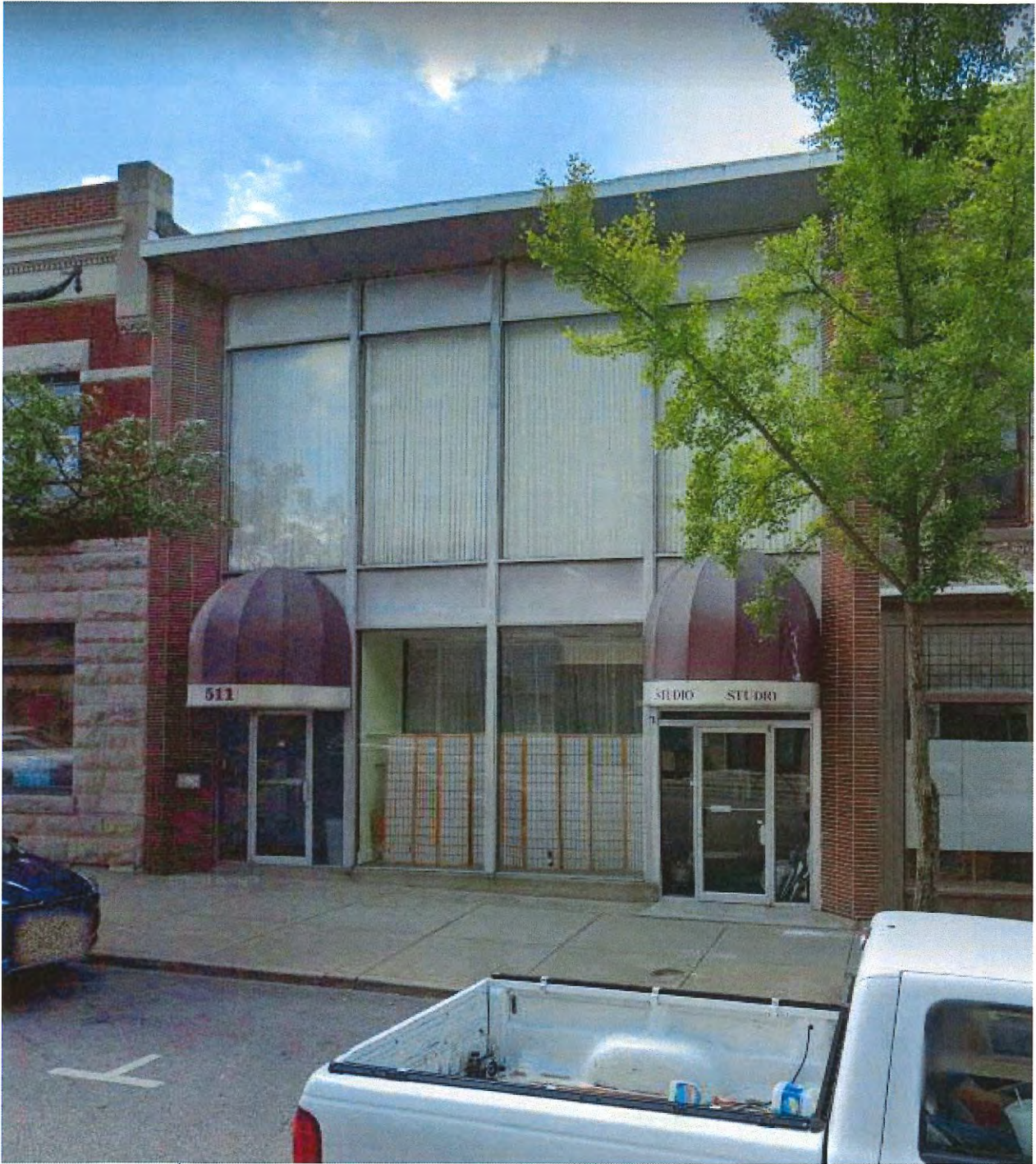
EXISTING CONDITIONS PRIOR TO 12/2/21 509-511 COLUMBIA ST.
